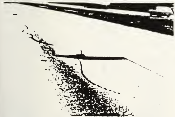
Fig. 3.2.4.2 — Meandering crack
